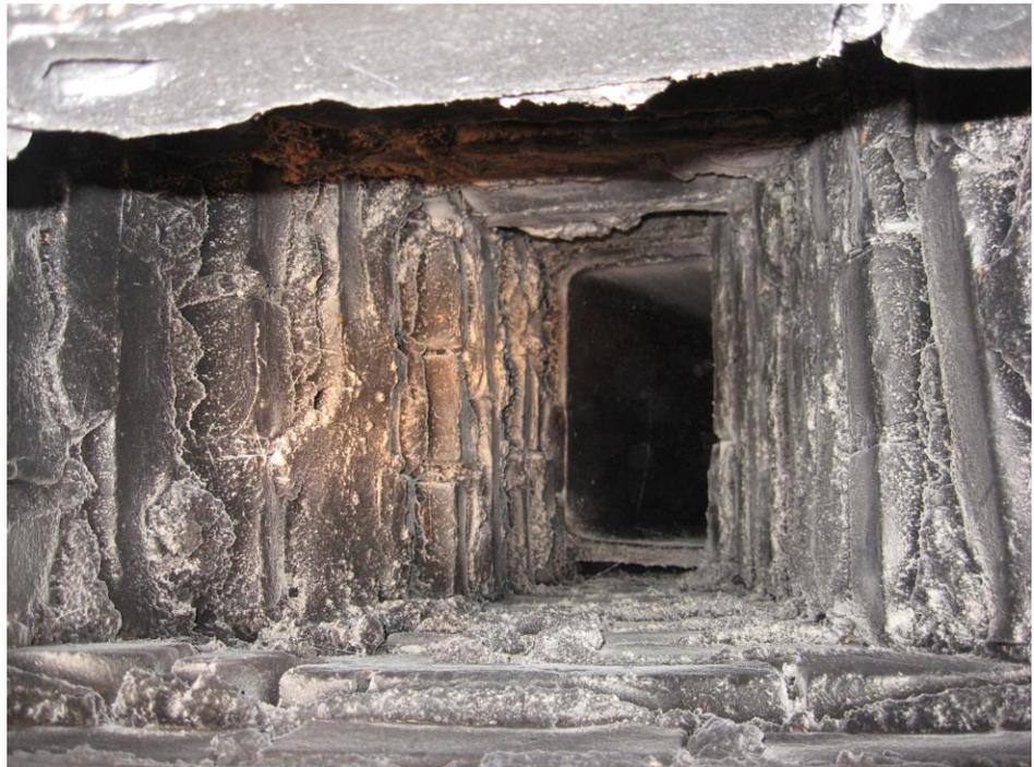
**Parging** is a type of stuccoing inside the chimney that is done for three main reasons. First, is to reduce turbulence in the flow of combustion gases. Second is to prevent combustion residue or smoke from leaking or accumulating in crevices or parts of the chimney. Third, it forms a uniform surface, since bricks and mortar can expand and contract with heat at different rates, that movement can create gaps. A single surface of like material lessens that risk.
