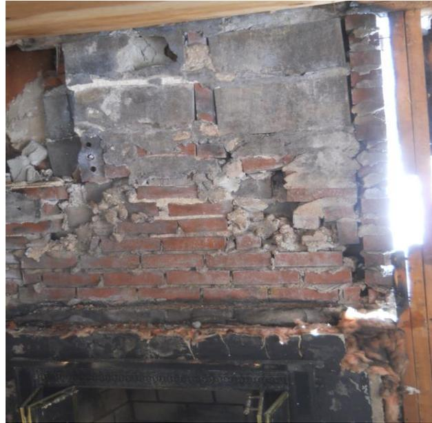
Therefore, when we repair an existing smoke chamber we use a specialized material that has insulative properties and is UL listed for **zero distance to combustibles**. The process usually involves removal of the old damper and frame so we can reach what is needed, hand forming of the material to form a single cast smoke chamber and the installation of a flue top type damper. Creating a finished product like the one to the right.
